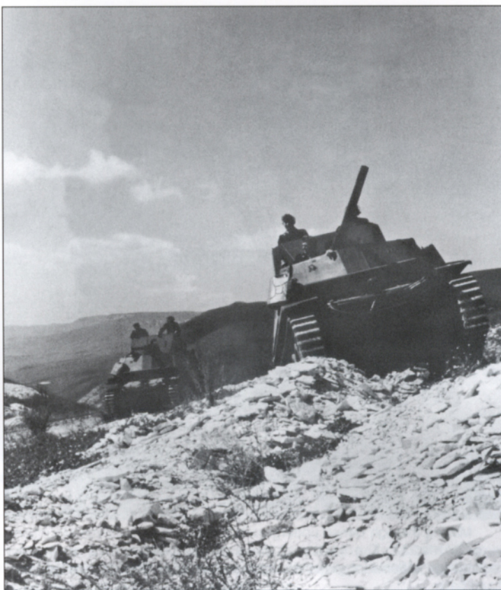
Unidentified vehicles of a Panzer-Division crossing the endless Russian steppes in the Don-bend area in July-August 1942. The tank is a Pz.Kpfw.III Ausf.J and armed with the new up gunned 5cm barrel.
